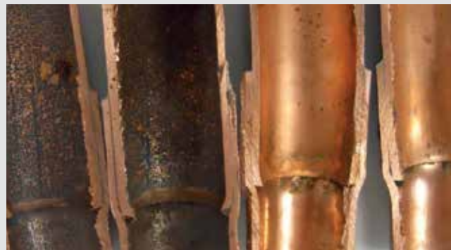
Without nitrogen purge
